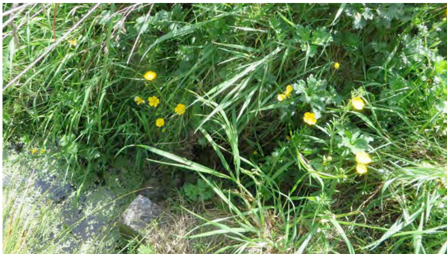
Photo 3: Water is flowing through the dam wall around the water control structure which is leading to wall failure.
