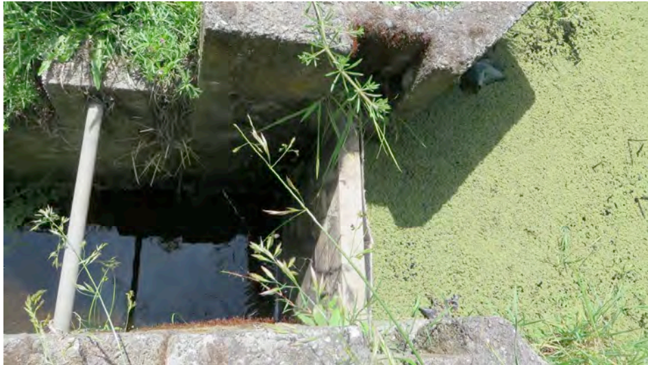
Photo 2: Water control structure on dam wall.
