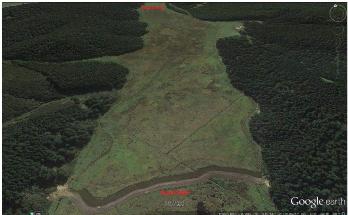
Figure 2: Position of new bund wall and approximate location of maximum water level when completely filled.
