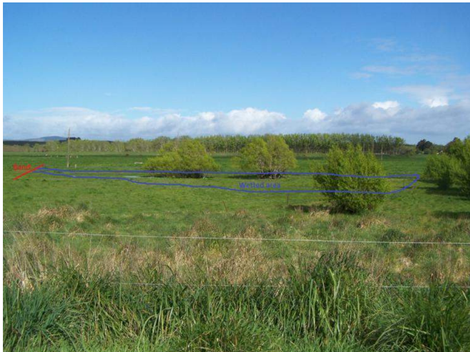
Figure 11: There is potential to create approximately 0.47 hectares of open shallow water by damming the outlet drain and swale
