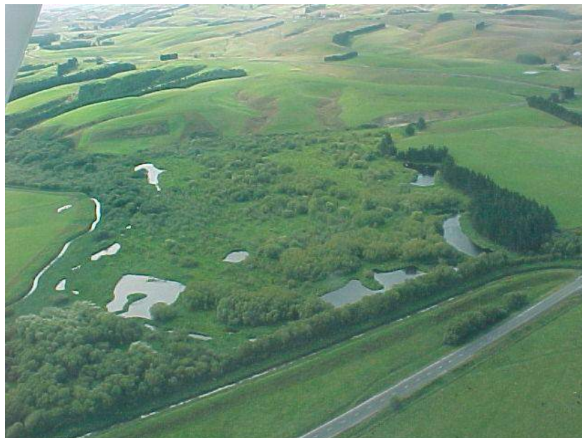
Figure 4: Waitepeka Wetland 31/1/2002, not long after the ponds had been excavated during high water table conditions and shows significant areas of surface water.
