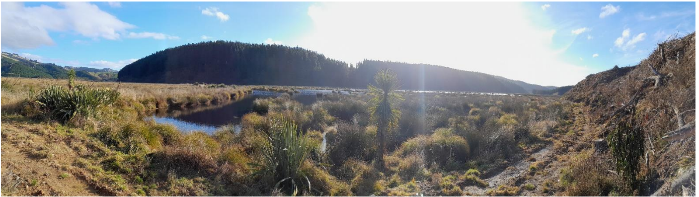
Bund wall and eastern culvert – June 2023
