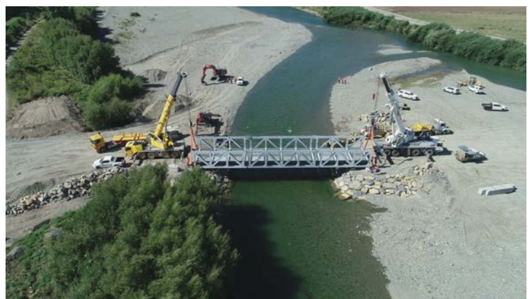
^ Temporary bridge over the Waimea River for carting gravel constructed by Taylors / Fulton Hogan
